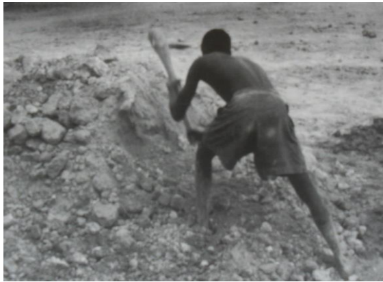
Fig.5(a) Preparing of reed mats, 5(b) Cutting of Azara, 5(c) Mixing of grass to Birji for strength, 5(d) Making of Tubali, 5(e) Excavation of Earth for making of Birji
