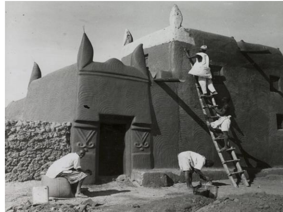
Fig.3(a) Traditional Hausa home under construction.
