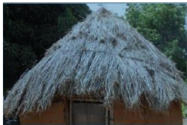
Fig.7(a) Typical Hausa Traditional building roof (Curvilinear conical design).[9]
